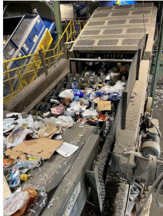
Figure 13 Material distribution on disc screen (Récup. Centre du Québec, Qc.)
