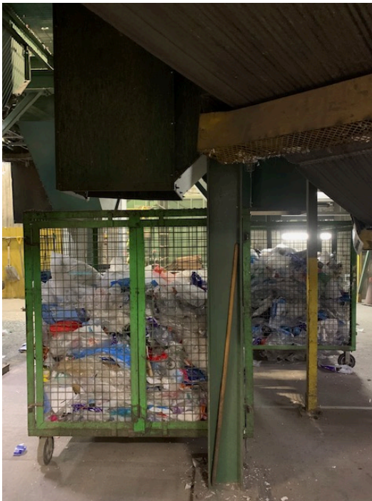
Figure 12 Storage equipment under sorting lines for manually removed FPP (Récup. Centre-du-Québec, Qc.). FPP was either sold to export or landfilled in 2022.
